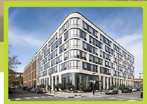
255 Brunswick Street - Hamilton House
