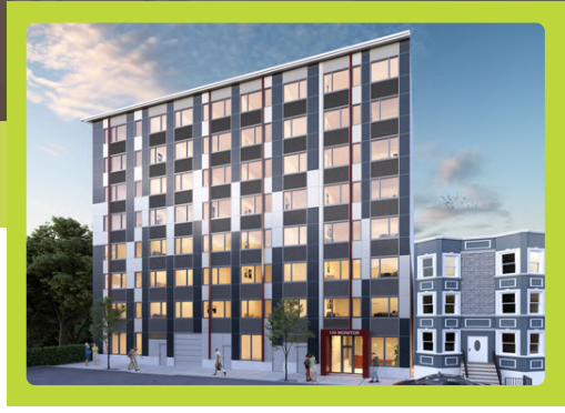
Under Construction - June 2025 Completion
