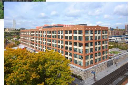
• Embankment House (250 Units - 1 Block)
