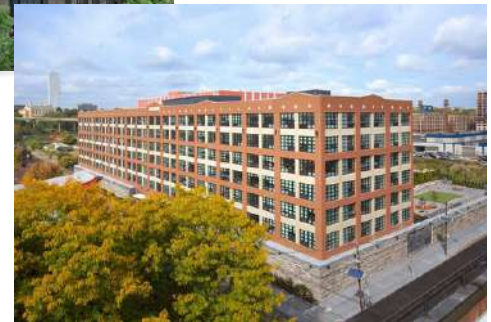
• Embankment House (250 Units - 1 Block)
